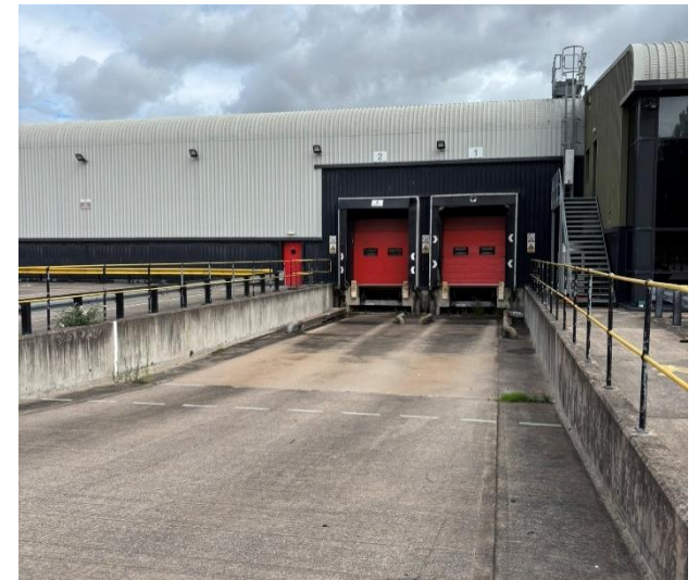
Warehouse Loading Docks
