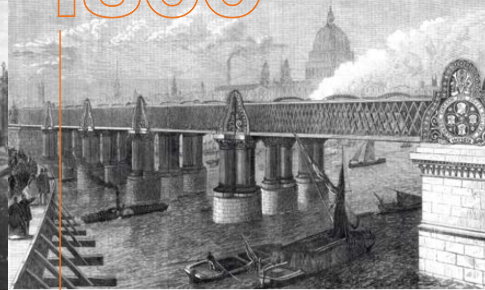
Blackfriars Railway Bridge constructed
