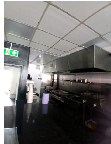
Kitchen and extraction
