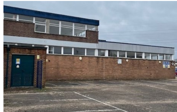
Secure gated yard
