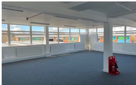
First floor office
