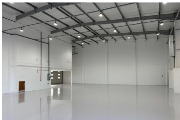
Indicative photo following refurbishment
