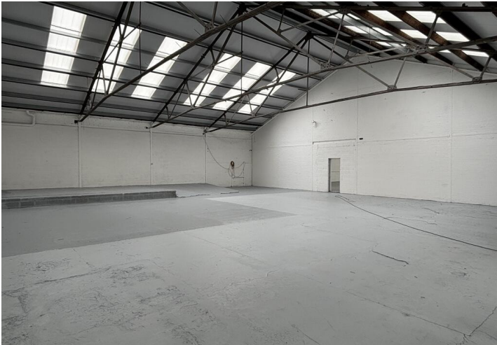
Refurbished warehouse accommodation
